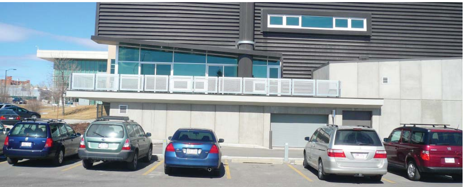
Parking in behind the Roderick Mah Centre for Continuous Learning
