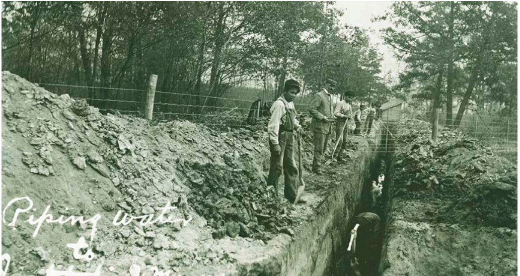
Children digging trenches for water pipes at the Mount Elgin Industrial Institute, Muncey [Mount Elgin Residential School], [circa 1909], file 90.162P/1169, United Church of Canada Archives, Toronto.
